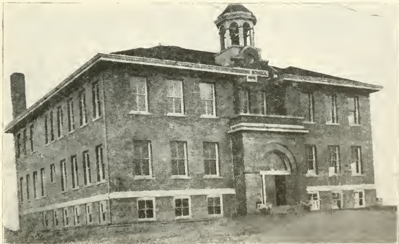
THE PRESENT SCHOOL, FAIRFIELD, BUILT IN 1906
